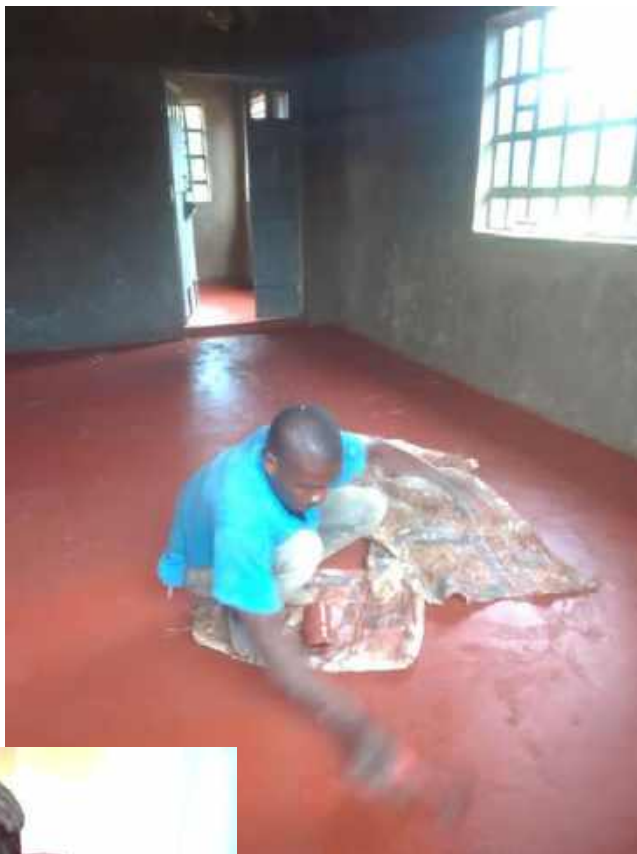
Electina's dilapidated mud house renovated with glass fitted to the windows, roof repaired, walls plastered, concrete floor laid and painted throughout.
